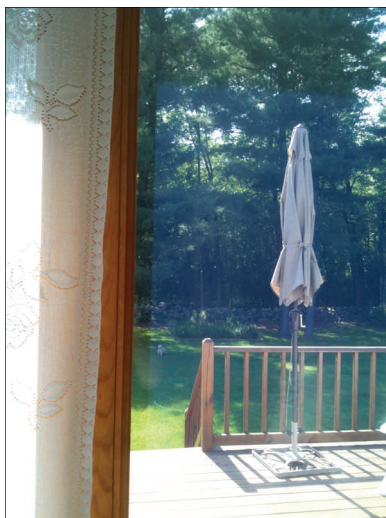
← “Haze” in Pilkington Energy Advantage partially sunlit area.
